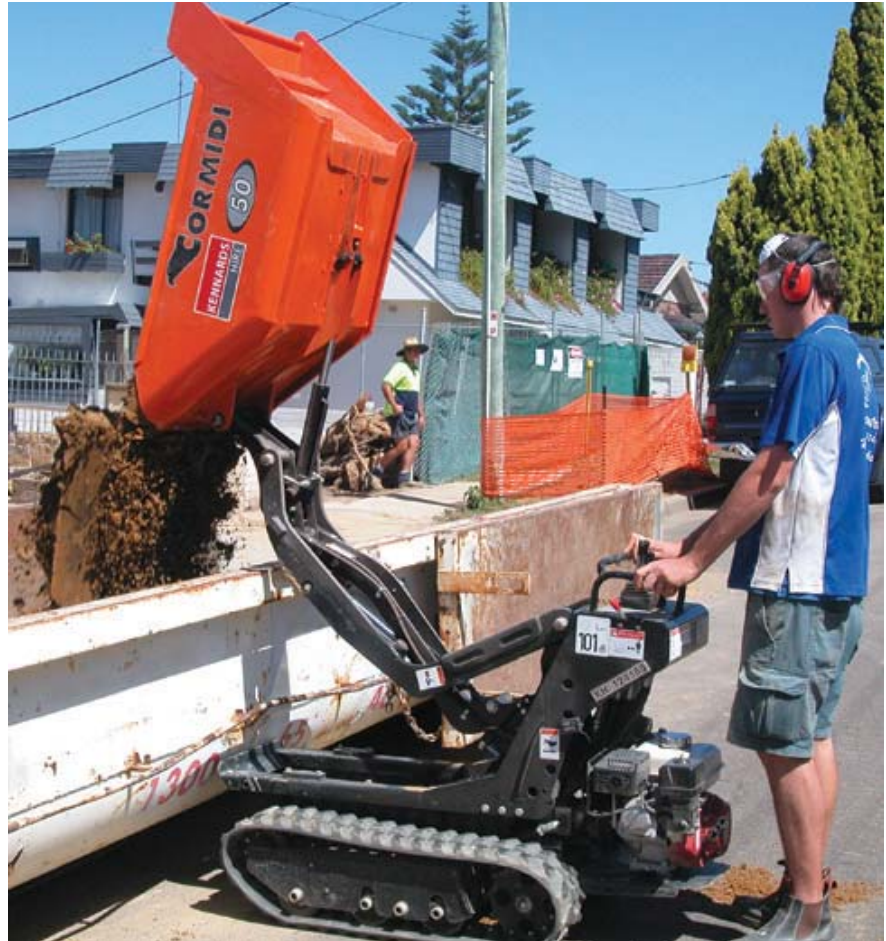
"Joey," one of the DB & HE Building Services team, moves a load of soil from the sub-floor excavation.
